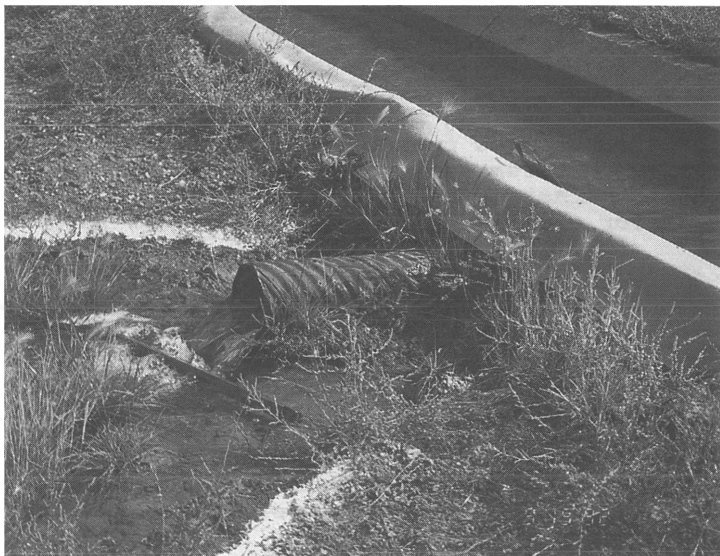
Fig. 1 Plastic lining of a concrete ditch
