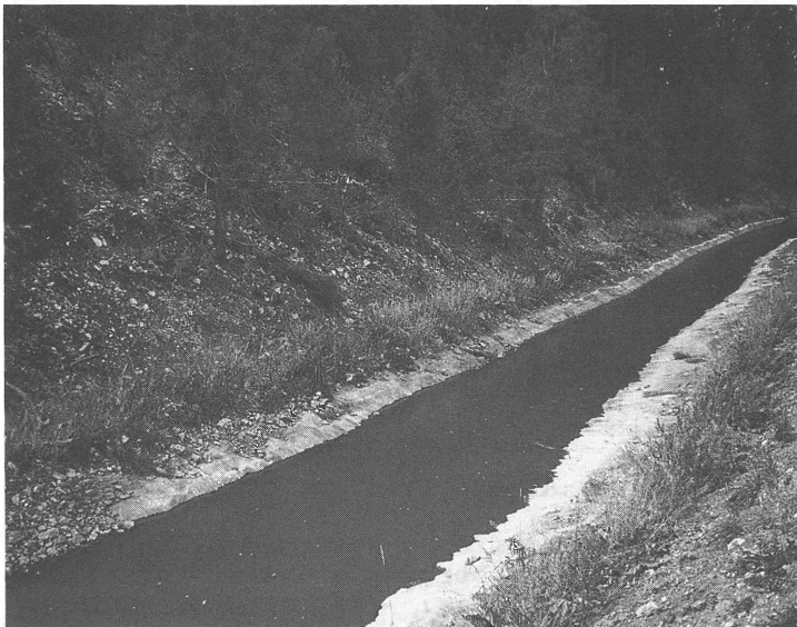
Fig. 2 Plastic lining of a rock/earth canal
