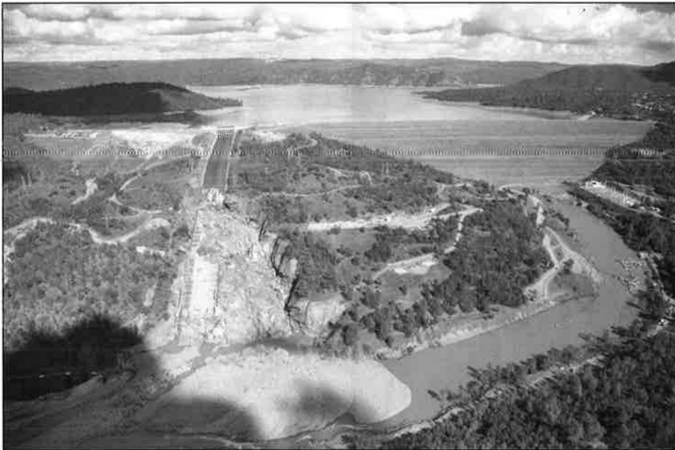
Figure 7. Oroville Spillway on February 27, 2017.
