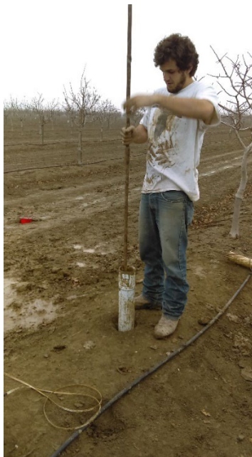
Figure 7. Polyethylene Septic System Pipe Used to Case 4" Auger Hole at Nees Farms
