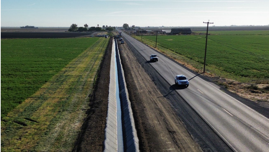
Figure 4. Completed canal section
