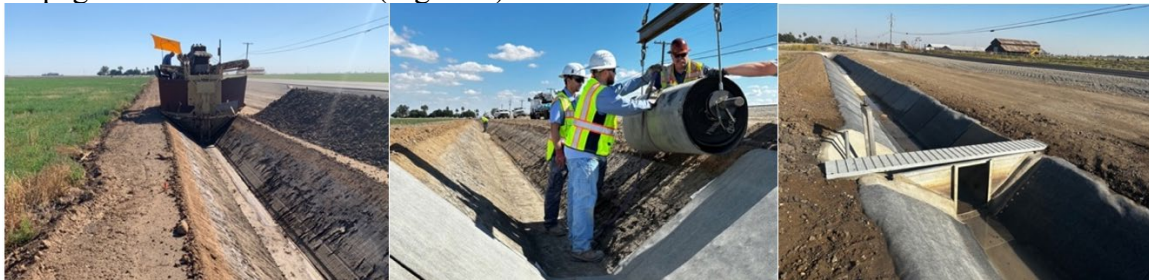
Figure 3. Reprofiling existing canal, deployment of GCCM and gates/valves.
