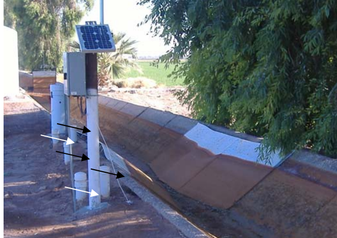
Figure 5. Venturi solution long-throated flume at MVIDD 18 & 19
