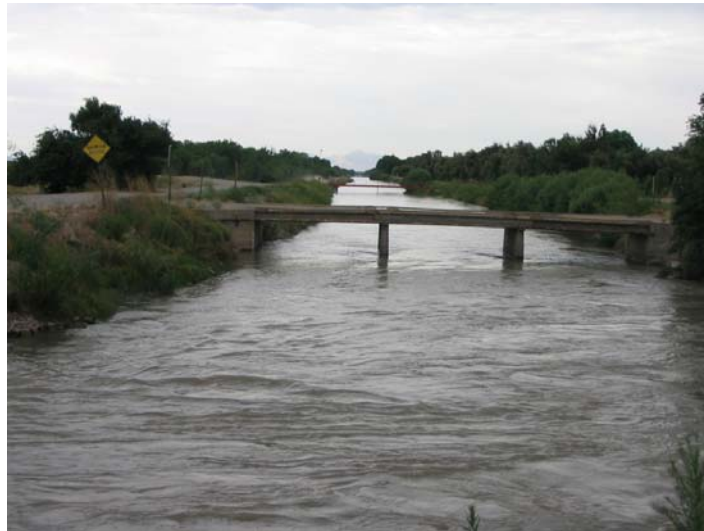
Figure 12. West Side Canal near the stream gaging bridge
