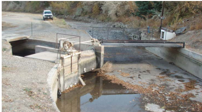
Figure 6. Photograph of the gate upstream of the chute
