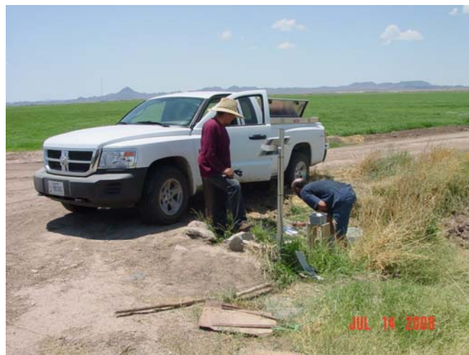
Figure 8. Installation of logging system at Palo Verde runoff venturi
