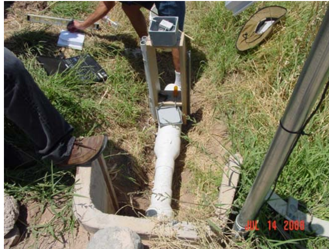
Figure 7. Runoff measurement venturi at Palo Verde
