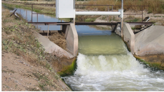
Figure 7. Fourth check on the Cochiti Main Canal
