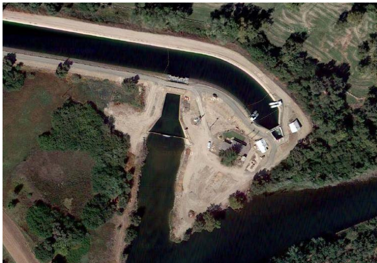
Figure 5. Kings River Siphon Hydro Project
