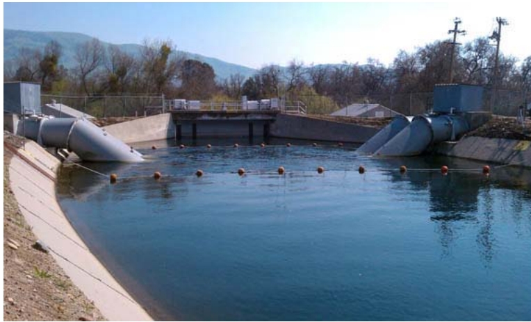
Figure 7. Intake from the Friant Kern Canal
