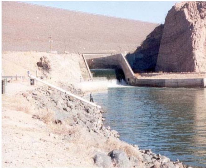
Figure 1. Cochiti Dam Outlet works, typical flow 28-42 m 3 /s, max. 200 m 3 /s
