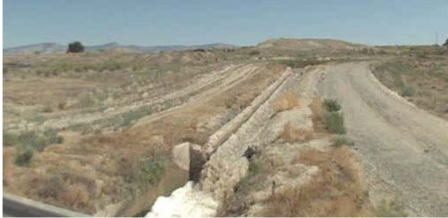
Figure 8. Photograph of the 18.5 Road Chute
