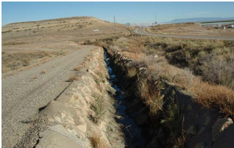
Figure 9. Photograph of the 13 Road Drop
