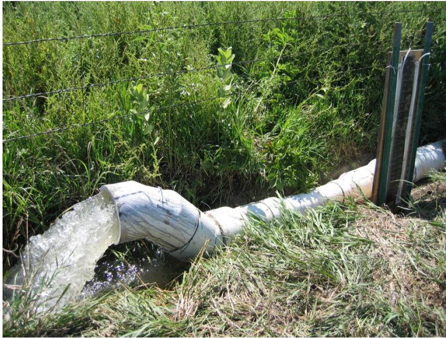
Figure 5. PVC Venturi meter and manometer installed at the second PID site
