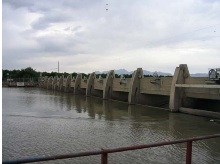
Figure 9. Upstream face of the Mesilla Diversion Dam
