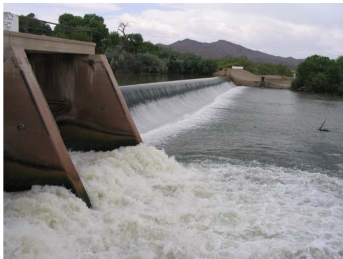
Figure 5. Percha Diversion Dam with radial gates in the foreground
