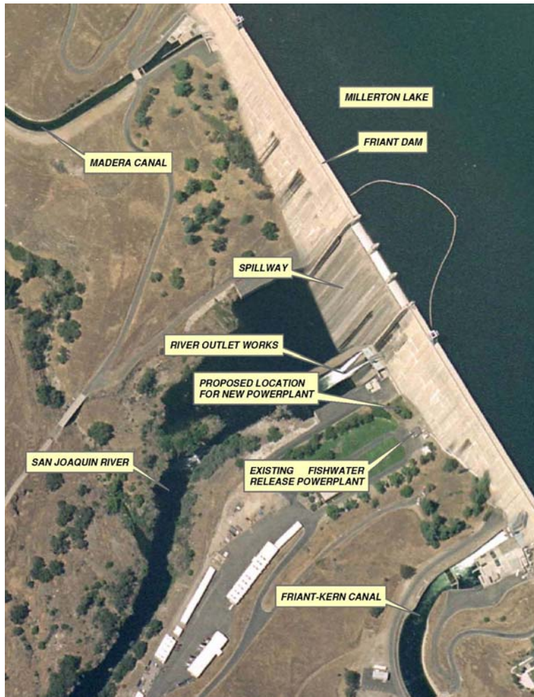
Figure 6. Friant Dam Facilities
