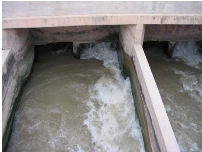
Figure 10. Turbulent flow under the sluice gates at the head of the East Side Canal
