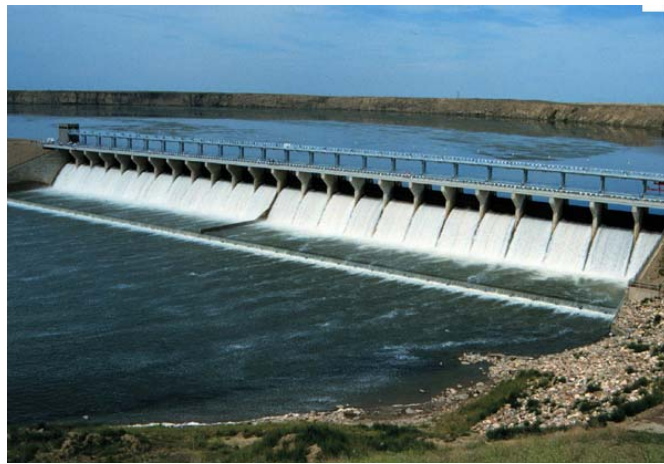
Drops at irrigation reservoirs or simple drop structures for energy dissipation can provide opportunities for energy recovery.
