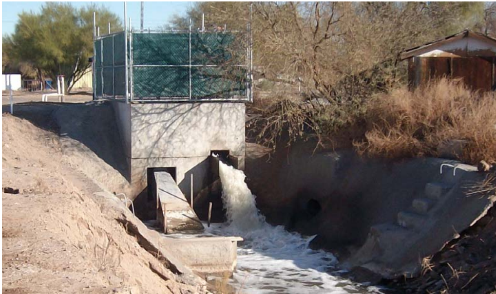
Figure 2. Installed vault prior to generator installation
