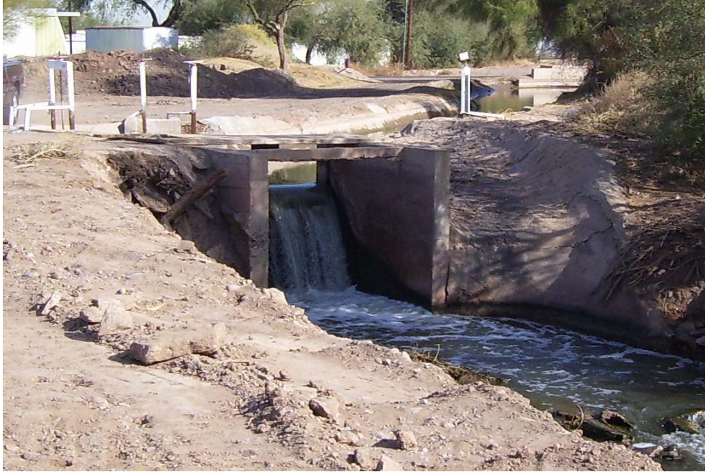
Figure 1. Original Drop Structure
