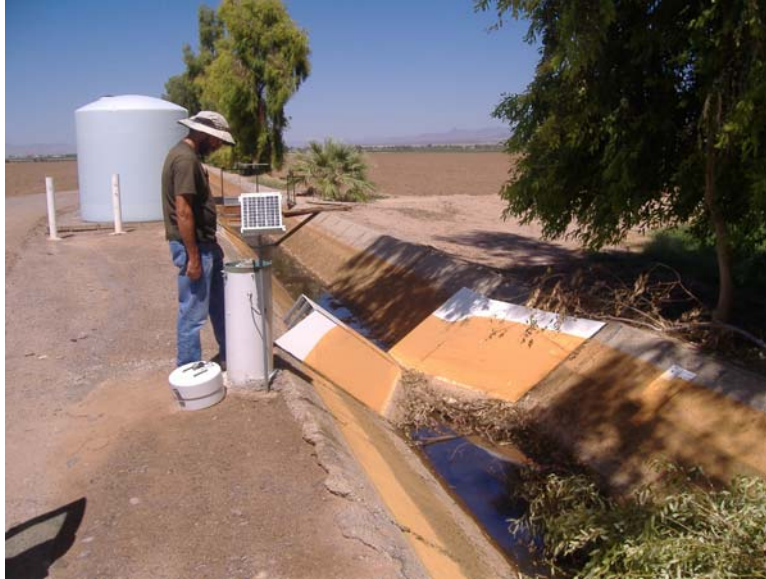
Figure 3. Open channel measurement field test at MVIDD wells 18 & 19 measurement site.
