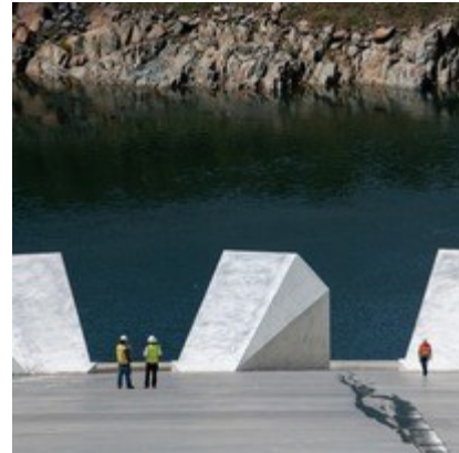
Routine Spillway Cleaning and Inspections Underway
