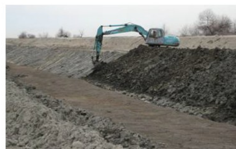
Figure 3. James ID Main Canal during side compaction
