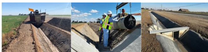
Figure 3. Reprofiling existing canal, deployment of GCCM and gates/valves.
