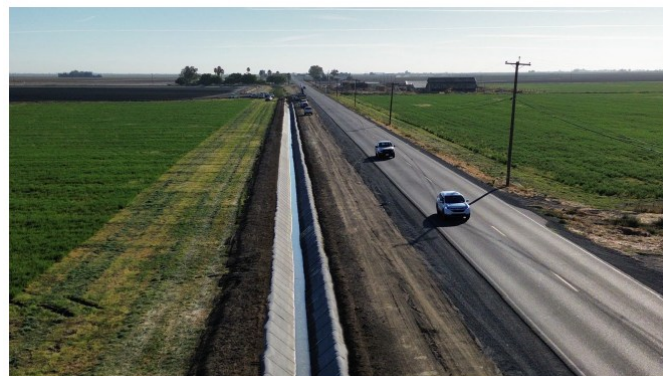
Figure 4. Completed canal section
