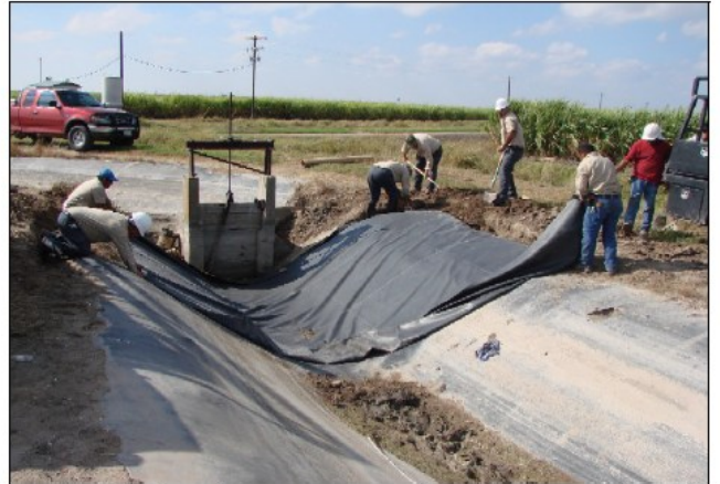
Figure 16. A district maintenance crew repairing a damage section of lining
